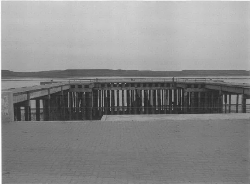
Vista general interior del Muelle
