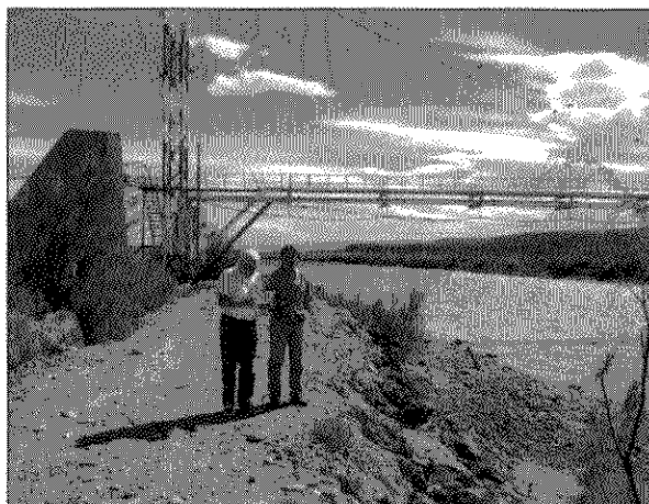
Pasarela Repsol YPF
